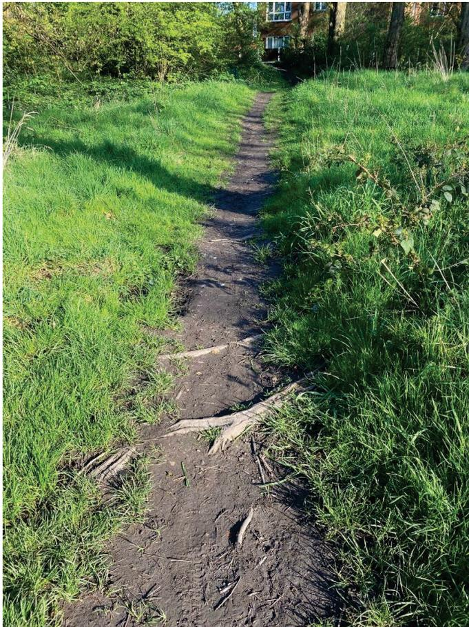
*Photo of path to be formalised with compacted aggregate. Tree roots to be retained and built over.*
